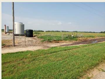
Figure 7: The downhill slope shows that the liquid fertilizer facility leading to the discharge area. The picture was taken on June 10 th
