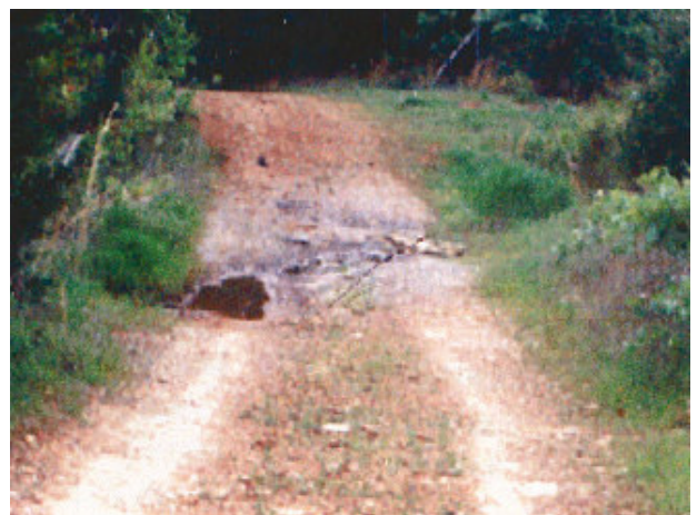
Figure 3a. This natural crossing on the Caney Mountain Trail can be improved with hand labor and local rock at very low cost.
