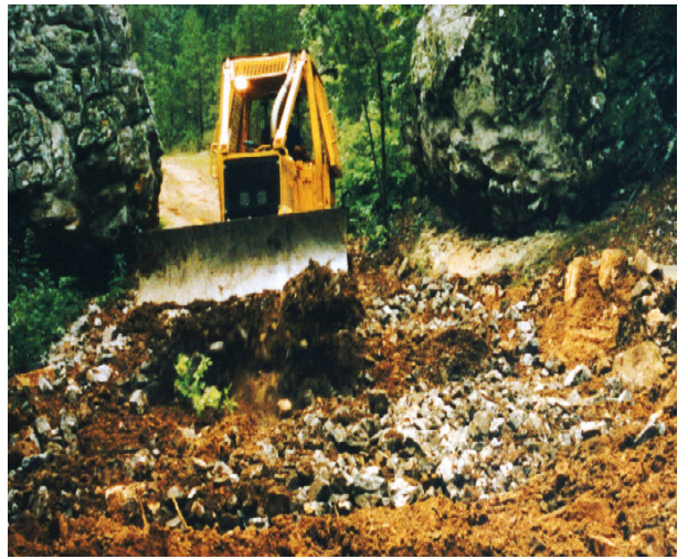
Figure 8b. Dozer filling channel with rock
