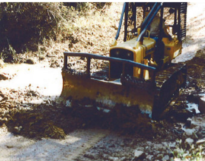
Figure 4c. The channel was excavated, then filled with rock
