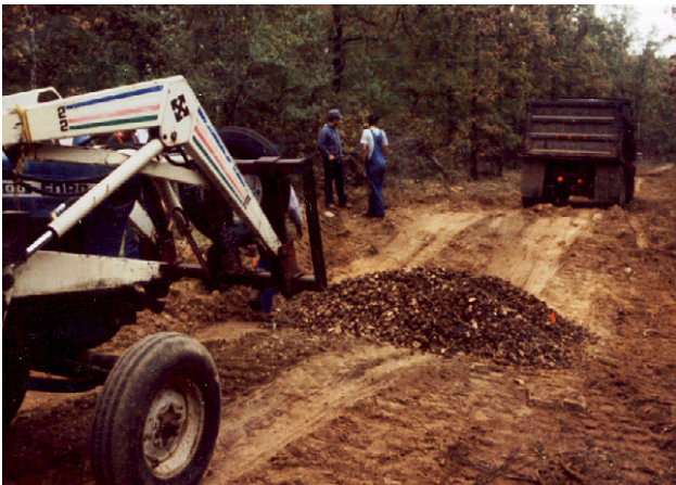
Figure 5. Placing a gravel fill in a ford on a light-use road
