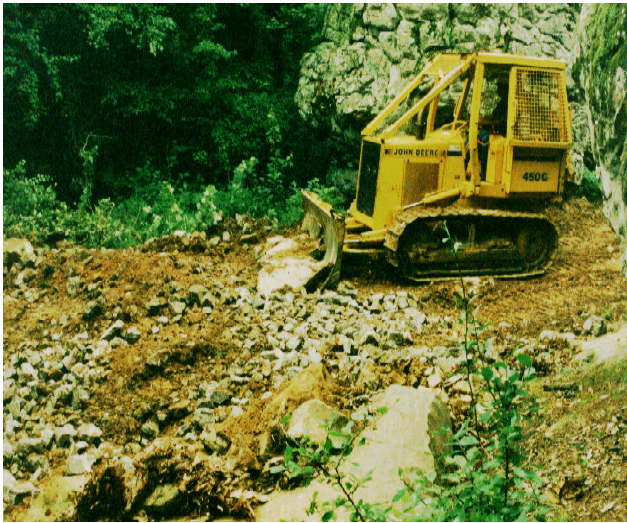
Figure 8c. Dozer pushing small boulder for end wall
