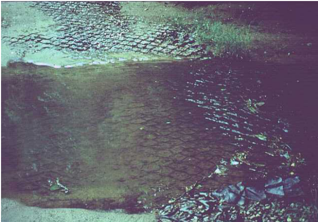
Figure 6. A Geoweb® and gravel fill surfaced ford
