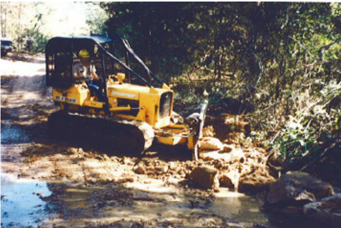
Figure 4b. Small boulders were pushed to build the lower end wall
