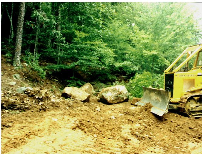
Figure 8e. Dozer placing large boulder flow dissipaters in channel above ford
