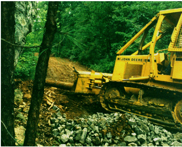
Figure 8a. Dozer removing old culvert and excavating channel
