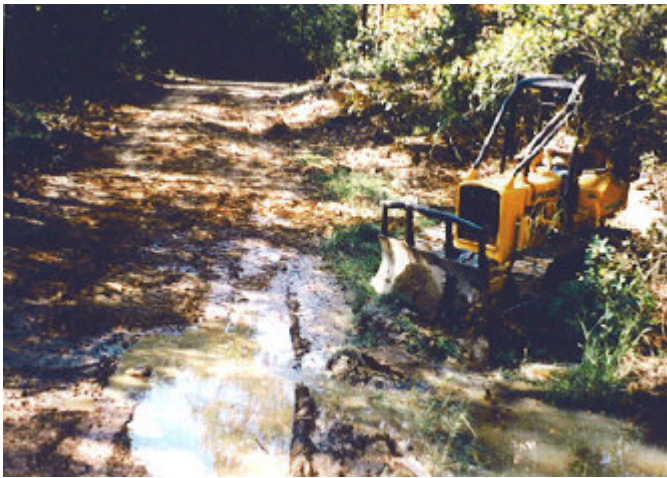
Figure 4a. This channel bottom is on deep soil and became a mud hole during log truck use
