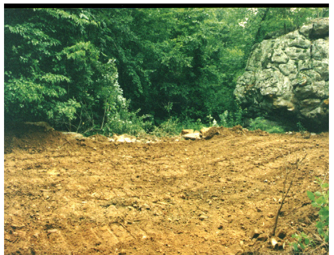
Figure 8f. Completed ford and berm
