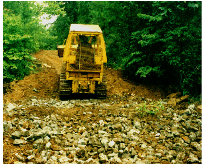
Figure 8d. Rock fill in channel and berm
