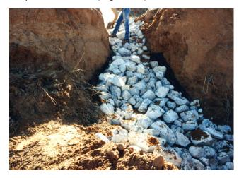
Figure 9b. Completed chute with large rock placed
