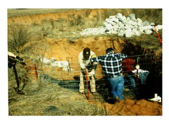
Figure 10a. Constructing the upper gabion
