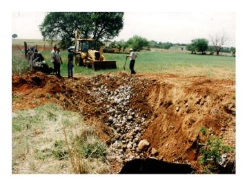
Figure 15e. Completed placement of rock
