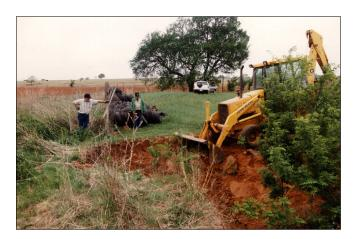
Figure 15a. First steps in construction on Example 3 were to shape and slope the upper gully area (note black locust saplings)
