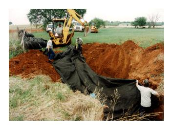
Figure 15c. Applying the geotextile fabric
