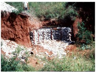
Figure 13b. Completed gabion drop-structure and apron
