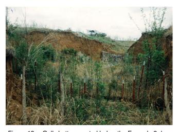
Figure 13c. Gully bottom control below the Example 2 dropstructure, constructed by placing cattle panels next to the gully sides and across the bottom. Photo was taken in the first growing season.
