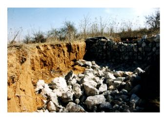
Figure 10b. Completed upper gabion and upper part of chute
