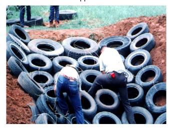
Figure 15d. Placing and wiring the tires
