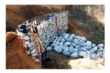
Figure 8b. Completed lower gabion with apron
