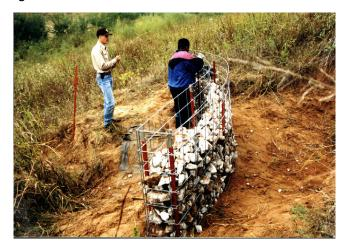
Figure 8a. Constructing the lower gabion drop structure
