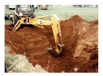
Figure 15b. The backhoe was used for final shaping
