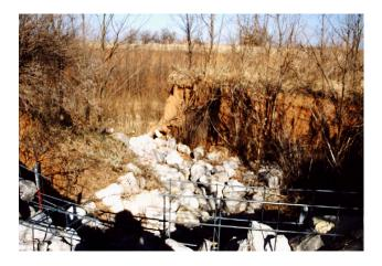
Figure 11c. Tree growth below upper gabion, in the first winter following treatment. The larger trees are 5 years old.
