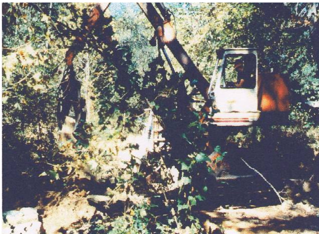
Figure 5. Log loader places boulders in Caney Creek ford end wall
