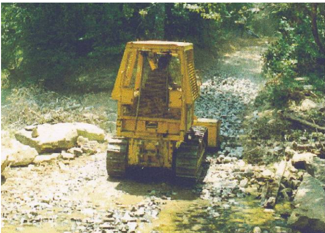
Figures 8a (above) and 8b (below). Rock surfacing of steep approach to the Caney Creek ford
