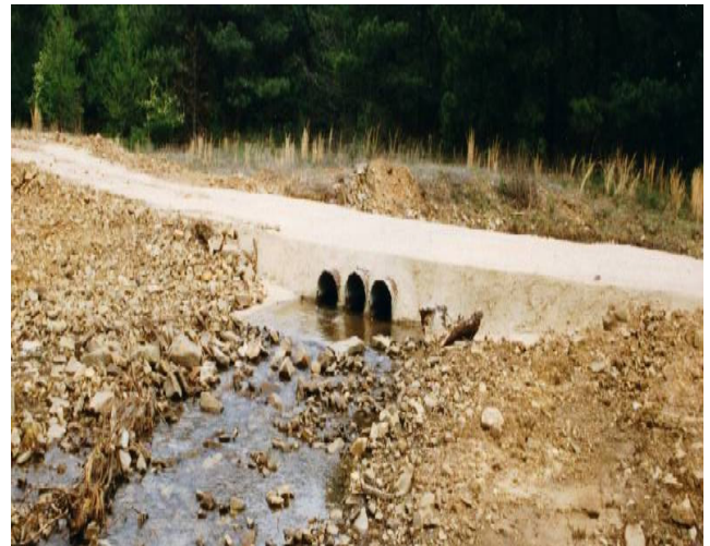
Figure 2. Vented concrete ford (slab)
