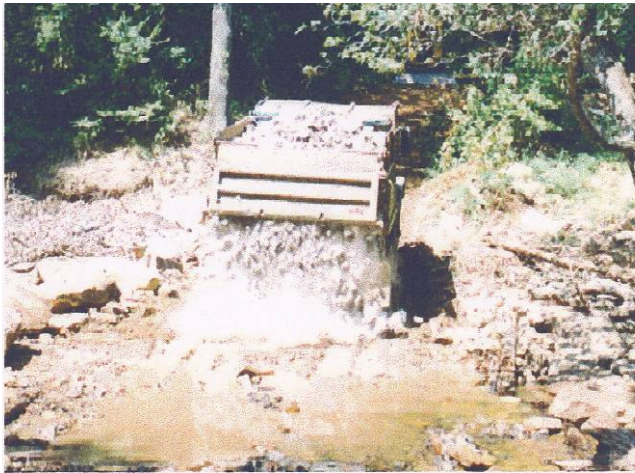
Figures 8a (above) and 8b (below). Rock surfacing of steep approach to the Caney Creek ford
