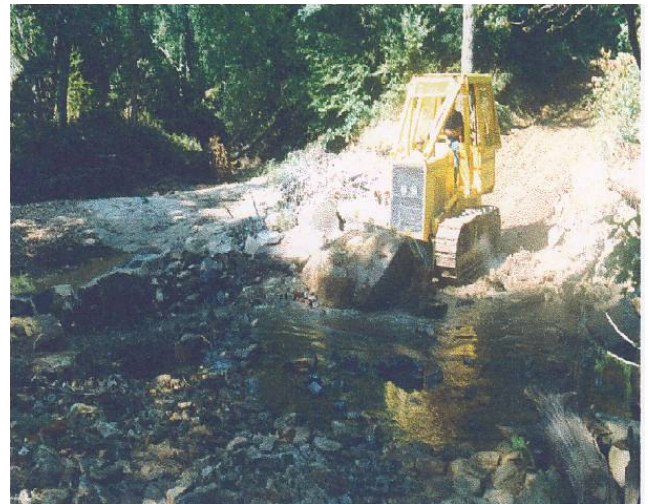
Figure 6. Dozer pushing and placing boulders on Caney Creek ford end wall
