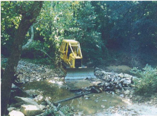
Figure 4b. Dozer beginning Caney Creek ford reconstruction
