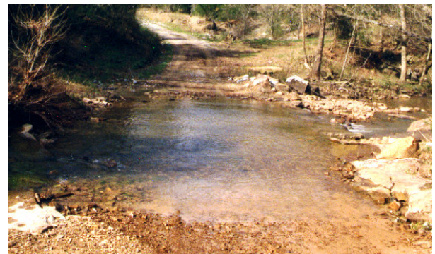
Example of well-designed rocky ford crossing
