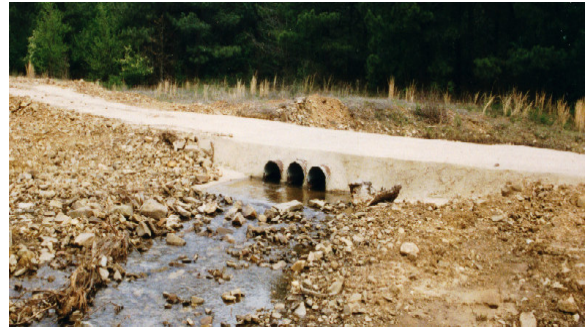
Vented concrete ford – a high dollar option.
