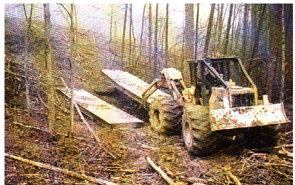
Temporary creek crossing "bridge mats"
