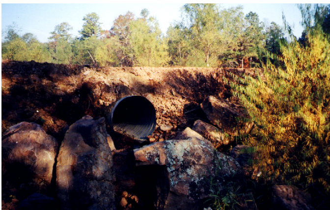
Large culvert in a road that crosses a small stream
