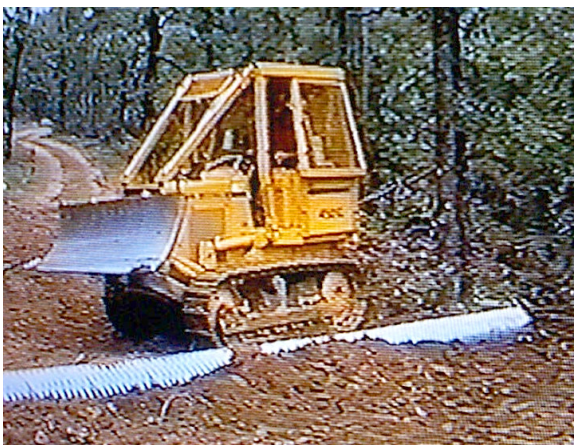
Figure 5. Tamping the fill using a dozer
