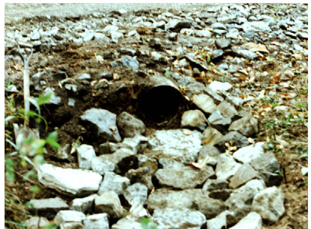
Figure 8. Where needed, place a rock apron below the outlet to prevent erosion.
