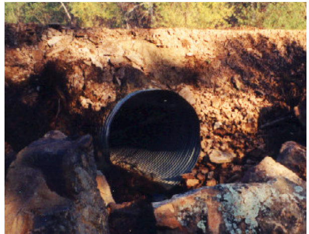
Figure 6. Depth of soil cover over the culvert is important to prevent damage
