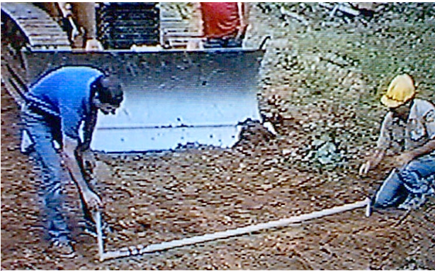
Figure 4. Using the shop-made Handy Gauge to measure a culvert bed slope of 3%
