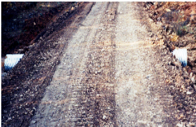
Figure 1. Properly installed culvert
