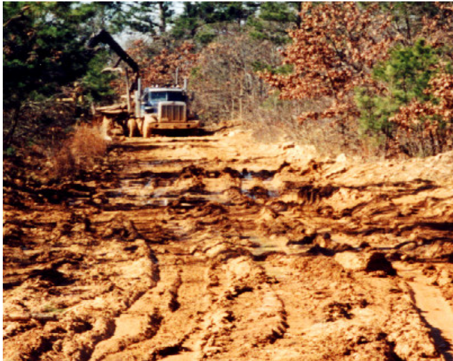
Figure 7. Ruts will develop quickly on roads with too little crown to provide good drainage.
