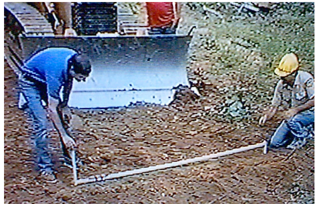
Figure 10. Measuring culvert bed slope
