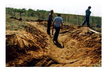
Figure 3. Planting seedlings after gully shaping and placement of fiber mat
