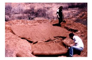
Figure 7a. Placing fiber mat in the second gully
