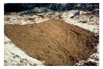
Figure 7b and 7c. Views of the completed fiber mat application looking upslope (Figure 7b above) and down slope (Figure 7c below)
