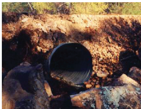
Figure 10. Cross-drain Culvert with Armored Outlet.
