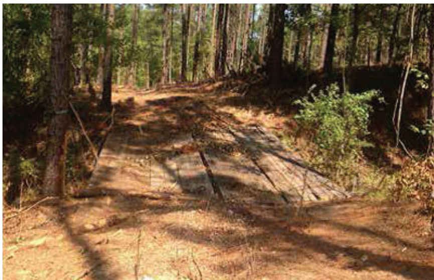
Figure 19. Portable Bridge Mats.
