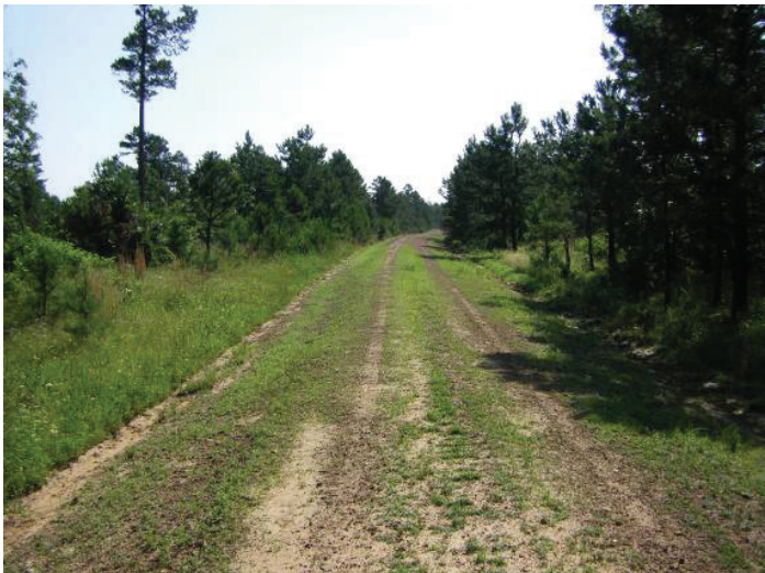
Figure 7. Crowned Road with Ditches.
