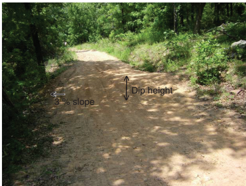
Figure 12. Example of a Rolling Dip.
